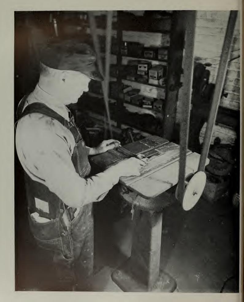
The Model A connecting rods are now on a saw table in which a rotating saw blade cuts the babbitt flange to complete the separating operation as shown in Picture 24. This also cuts the necessary oil relief groove through the flange.
